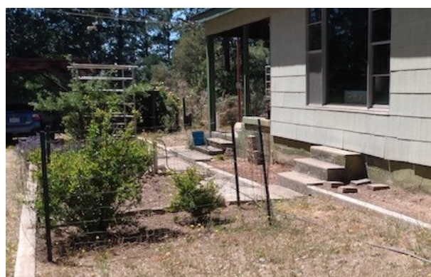
Another home assessed in Oak Hill area, showing great clearance 5 ft from house, and noncombustible foundation for first foot up.
